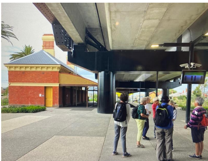
Moreland station – alongside the original station buildings
