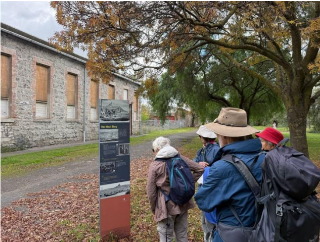
The Melbourne Meat Preserving Company preserved and canned meat in these bluestone buildings.
